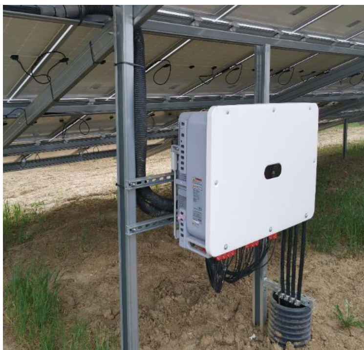
Fig. 7 – Inverter montato in campo
